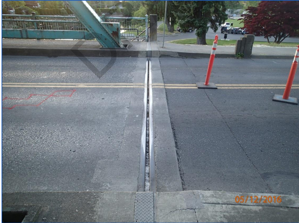
Photo 20: Fixed joint at the east abutment facing north.
