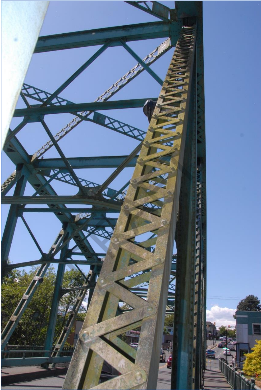
Photo 53: Oblique view of diagonal brace, west side.
