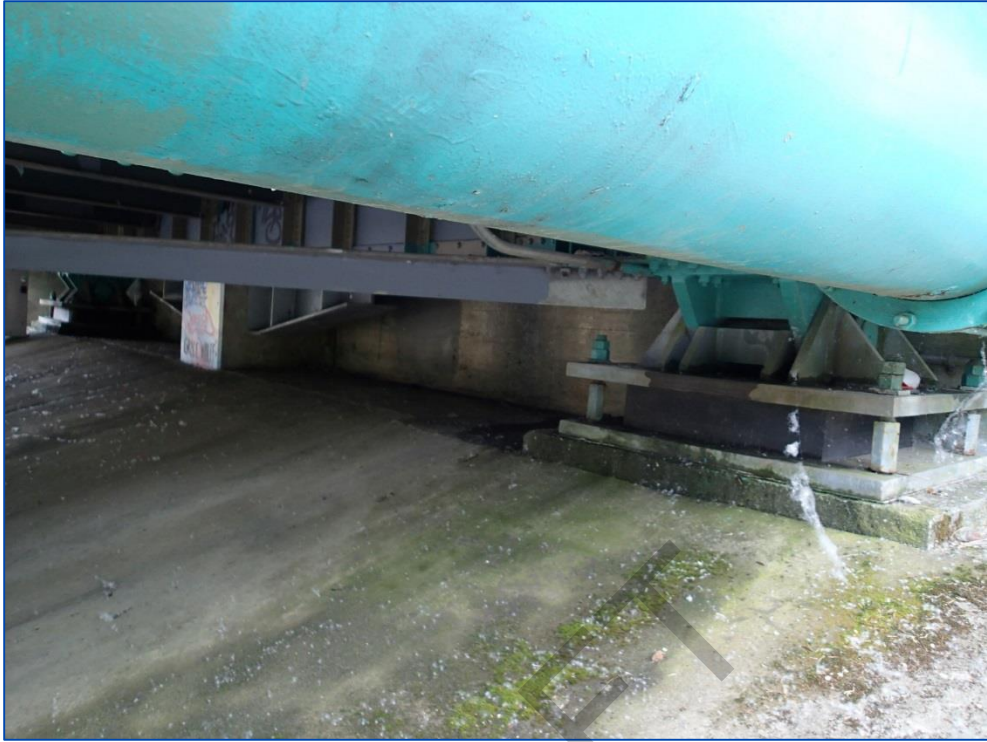
Photo 39: South bearing of east abutment.
