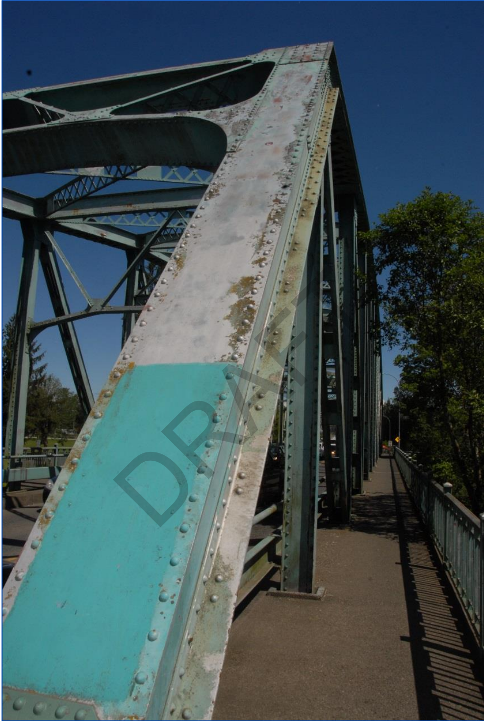
Photo 46: Oblique view of top chord at southeast corner.
