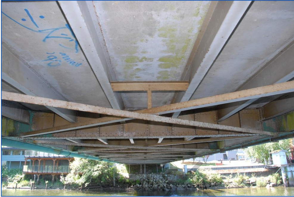
Photo 57: General view of deck framing as seen looking south.
