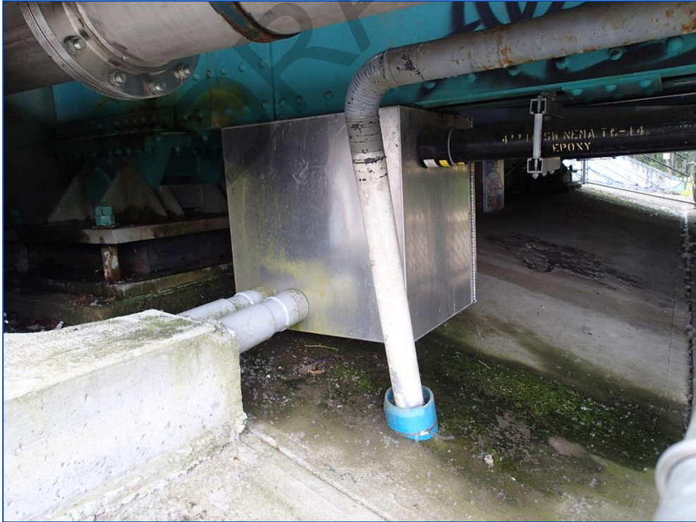
Photo 38: East abutment facing south.
