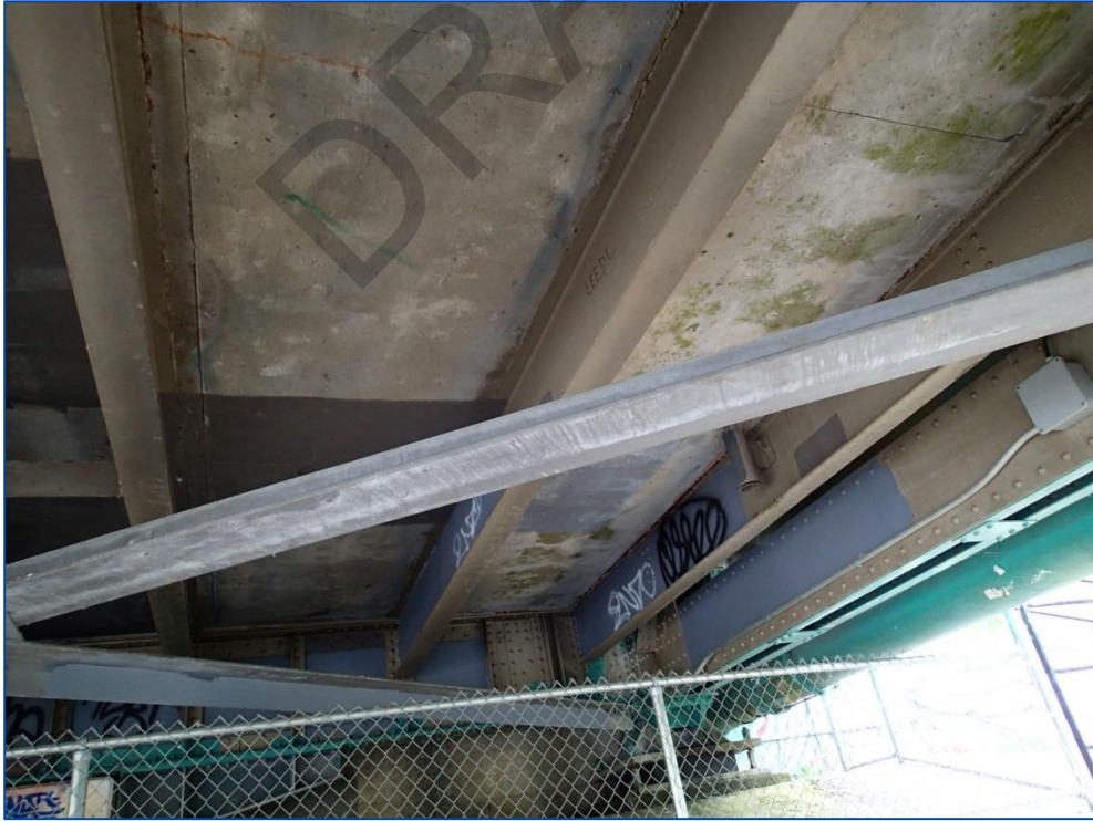
Photo 34: Southern half of deck soffit and sidewalk near the east abutment.
