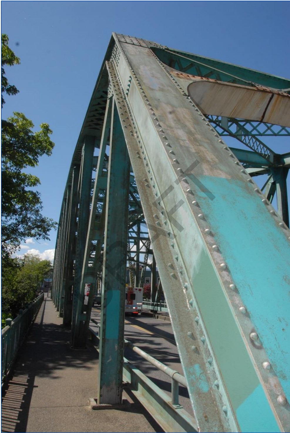
Photo 47: Oblique view of top chord at southwest corner
