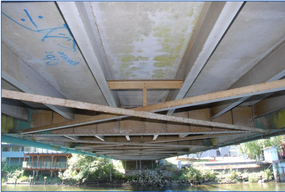
Photo 23: Structural steel and deck soffit between the river shores facing west.
