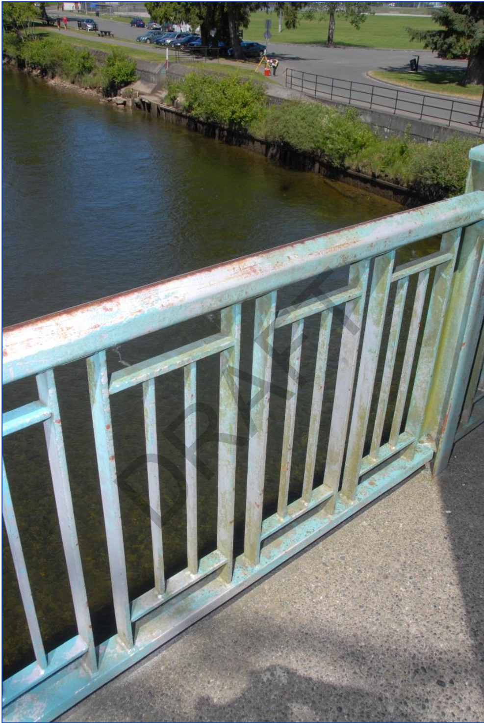
Photo 56: Typical pedestrian railing, east (downstream) side.
