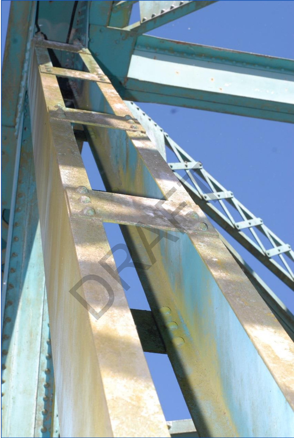
Photo 52: Oblique view of diagonal bracing in truss, east side.
