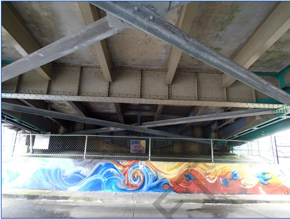
Photo 37: General view of the east abutment.
