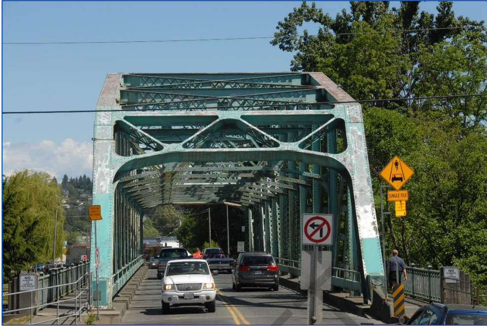
Photo 45: General view of south end.
