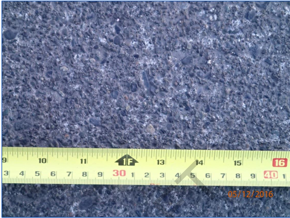
Photo 13: Close-up of deck surface showing minor loss of paste (typical).
