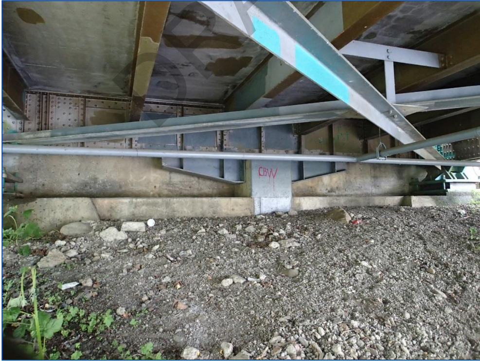
Photo 36: General view of the west abutment.
