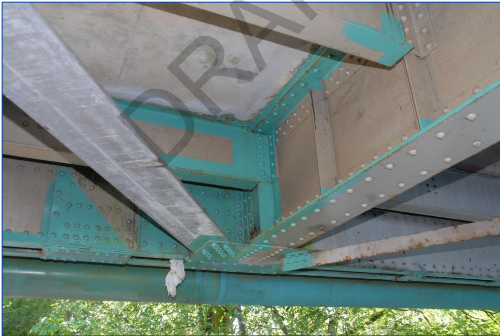
Photo 58: Typical touch-up coating, east side
