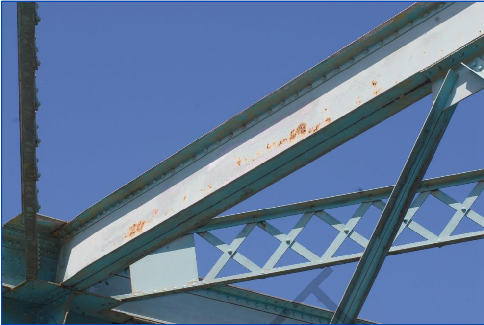
Photo 48: Typical transverse bracing near southwest corner of bridge.
