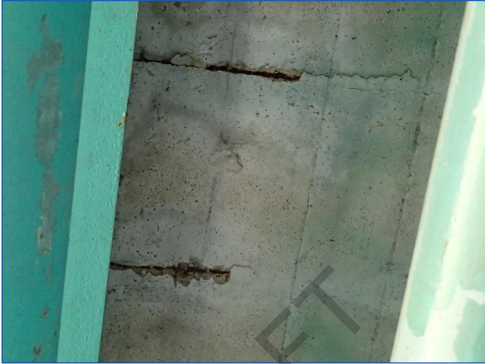
Photo 31: Close-up of Photo 30.
