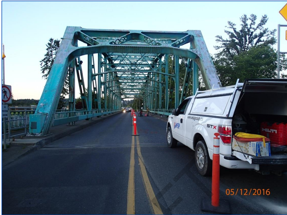
Photo 3: Deck view facing east.
