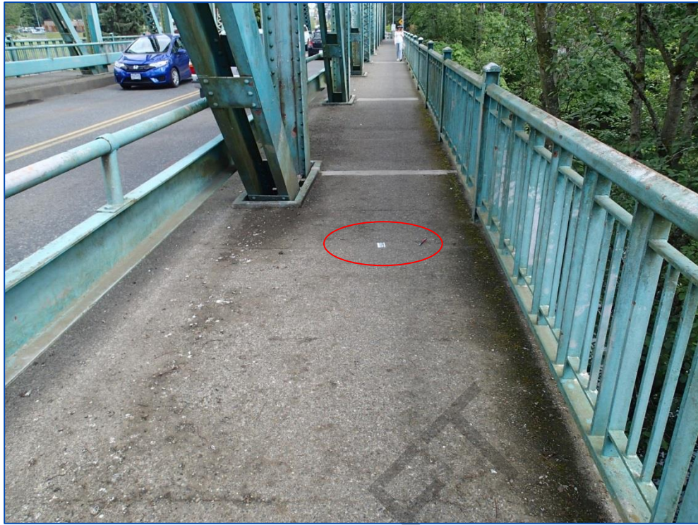
Photo 15: South curb and sidewalk facing east.
