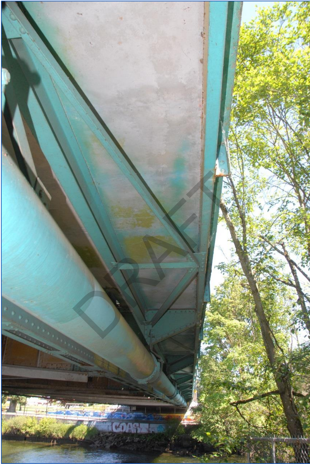
Photo 60: East side soffit below deck.
