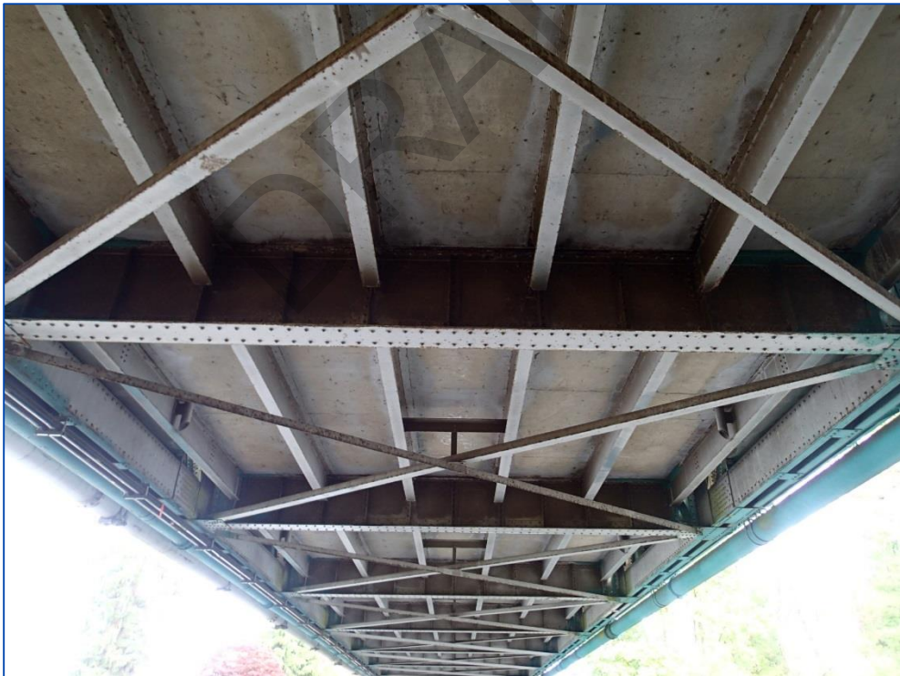
Photo 24: Structural steel and deck soffit between the river shores facing east.
