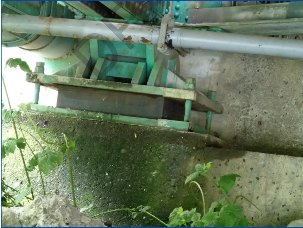
Photo 40: South bearing of west abutment.
