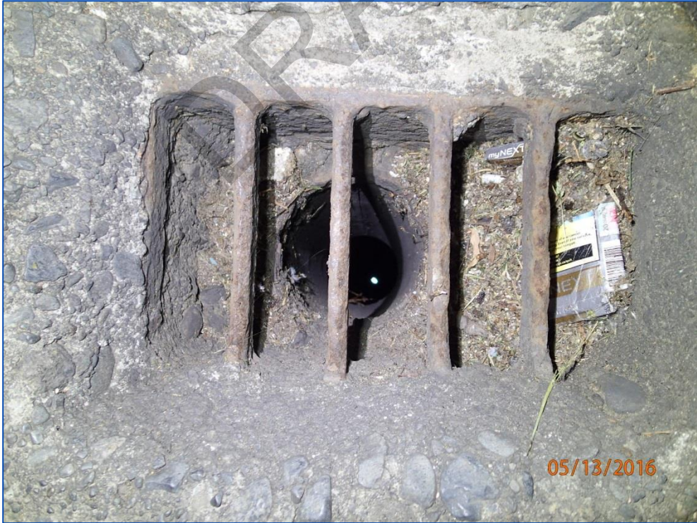
Photo 18: Condition of the drain (typical).
