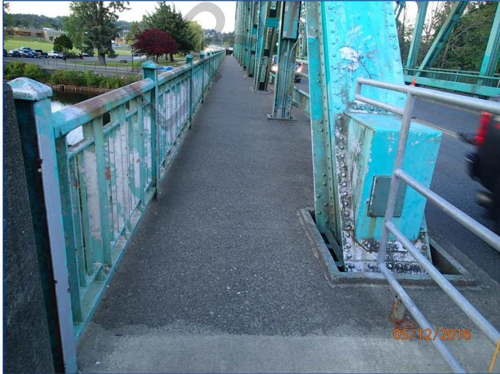
Photo 14: North curb and sidewalk facing east.
