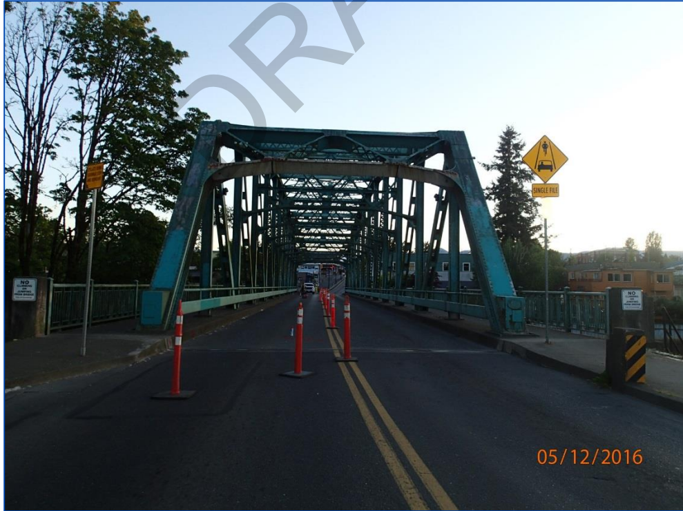
Photo 4: Deck view facing west.
