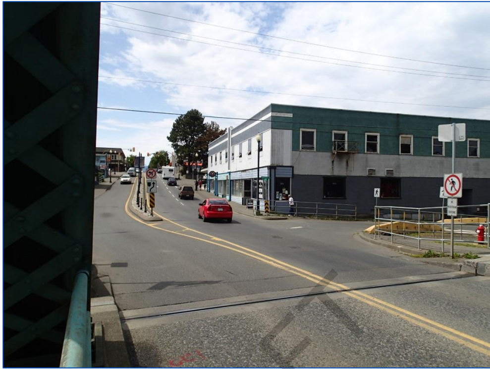
Photo 21: West asphalt approach.
